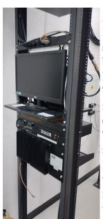
As shown in the picture on the left, the repeater is mounted in a standard equipment rack. The bottom open space is where the RF cavities are normally mounted. This picture was taken after their removal. The unit at the bottom (as shown) is the RF amplifier. The amplifier being used now is not owned by our club. It is "on loan" from CCFLARES. As a club we are looking for an amplifier to replace the CCFLARES unit. Fortunately CCFLARES knows this and are willing to support us until
